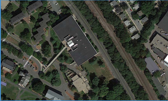
Dowling Hall Garage
