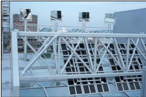
**Roof mounted mirrors, heliostats, direct light into the building through a skylight.**
