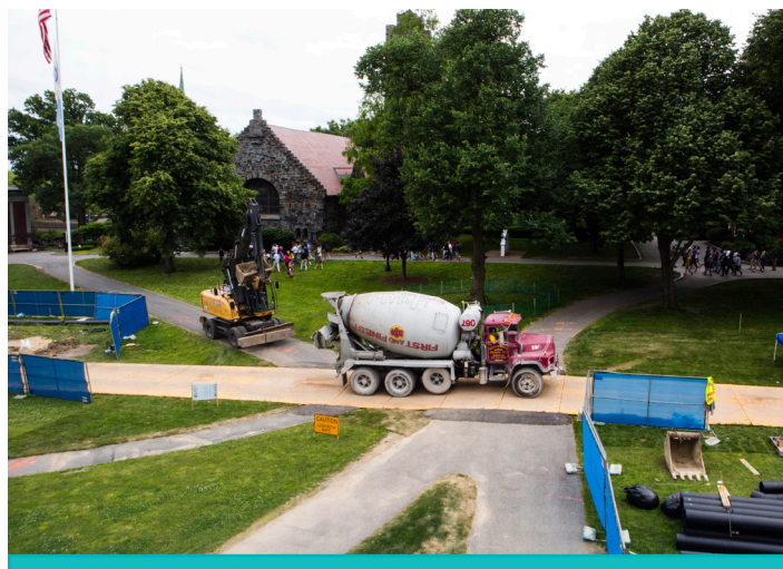
Pipes being installed to deliver chilled water from the Central Energy Plant to campus buildings.
