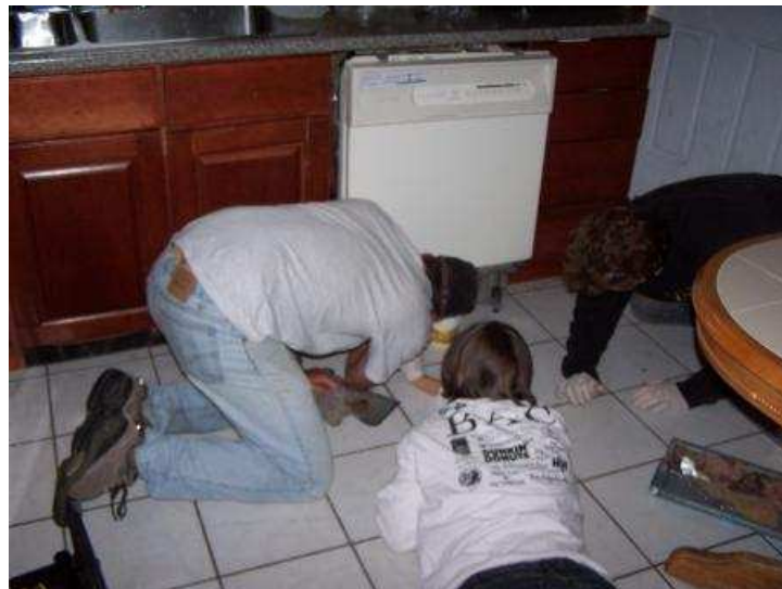
Tina tries to be helpful in the efforts to remove a dishwasher in order to airseal the holes in the wall behind it at a September 2009 HEET barnraising.
