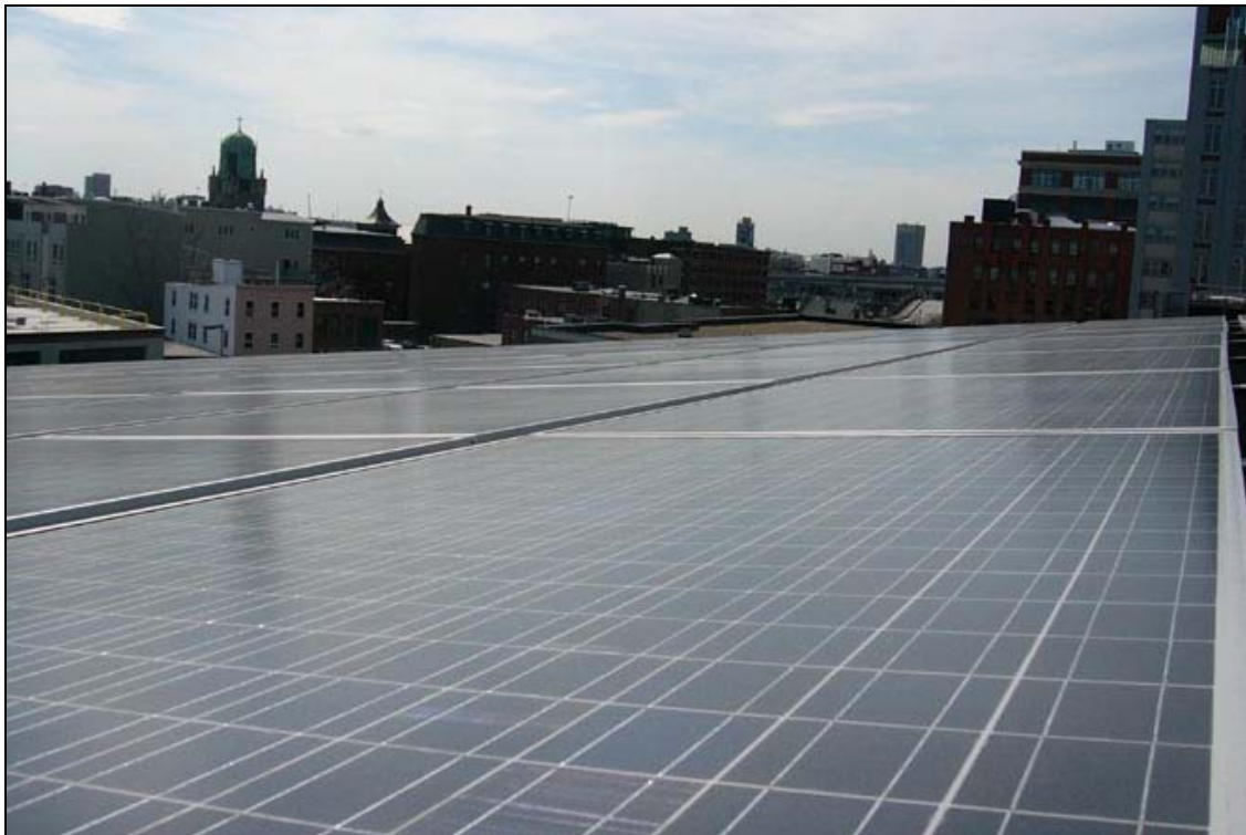
AFH's 42 kW PV roof array
