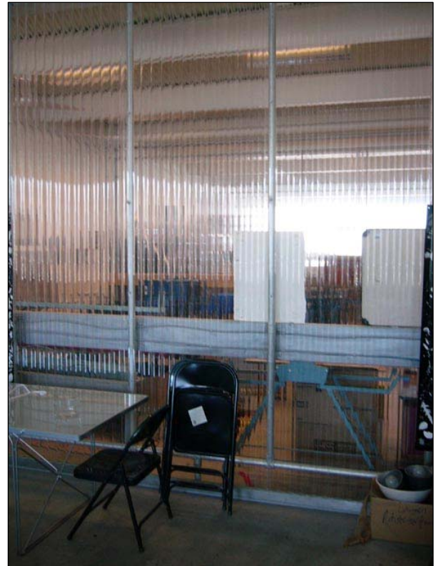
Creative use of low-cost building materials: Plumbers pipe is used to hold up the transparent dividers between studios.
