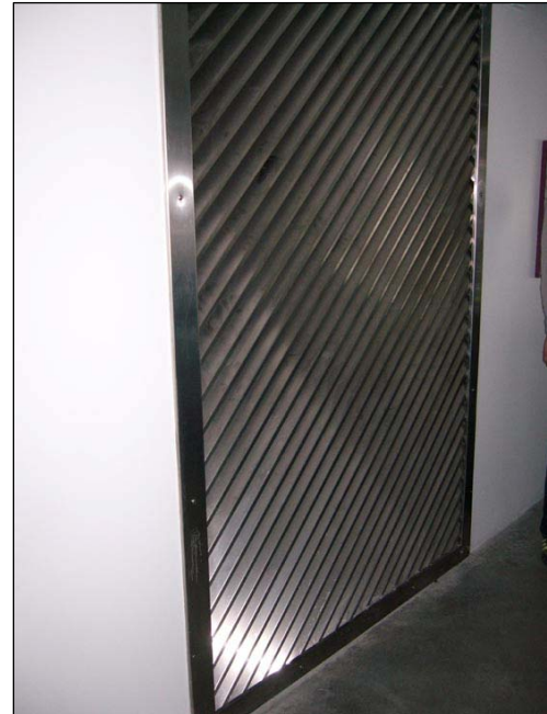
Cooling Tower Air Grates
